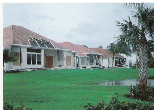
Gone with the wind screens destroyed on 3 Romora Bay houses photo by Helen Tator
